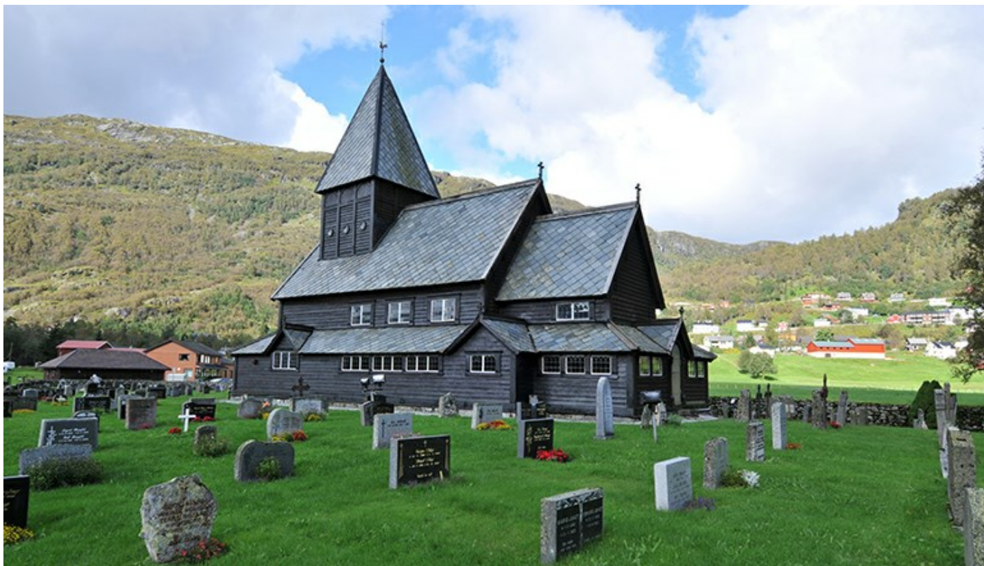
Røldal stave church in Odda in Hordaland county. Photo: Leif Anker, the Directorate for Cultural Heritage
